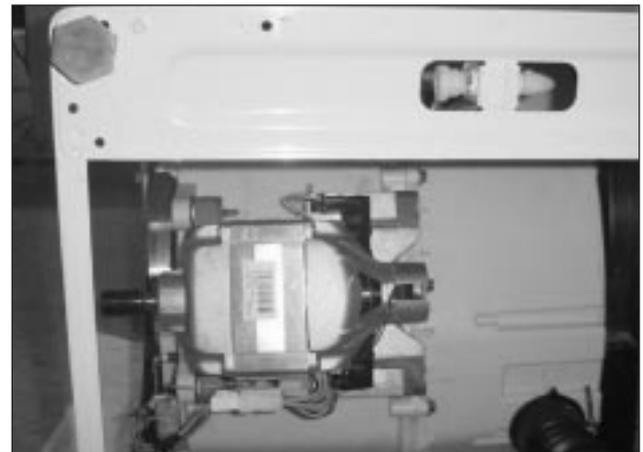
3) Remove two bolts and two nuts mounting the motor by using a box wrench.
